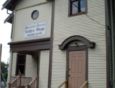
4519 S. Claiborne - former rectory
